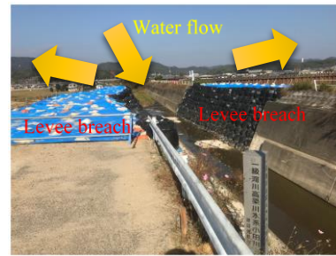
Fig. 2 Levee breach at Oda river in Mabi City (The first author took the picture on November 10, 2018)
